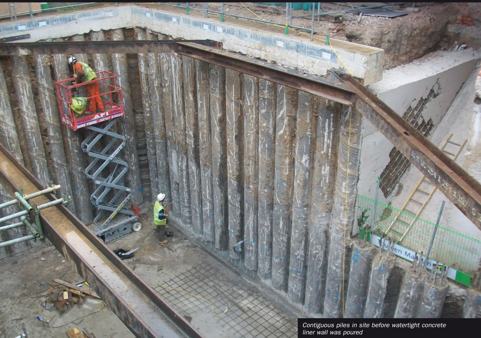
Contiguous piles in site before watertight concrete liner wall was poured
