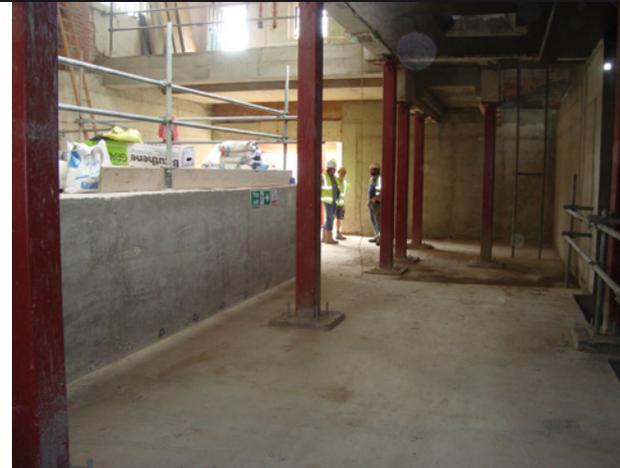
*300m<sup>3</sup> of watertight concrete have been used to construct the new basement beneath and beyond the original building*
