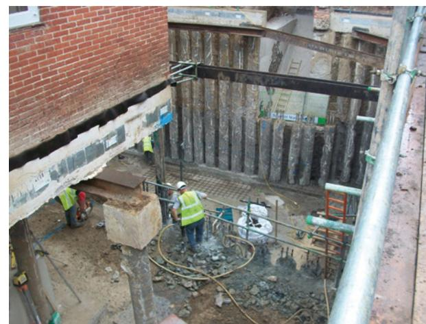
The original house sits on top of RSJ props while the new basement is excavated below
