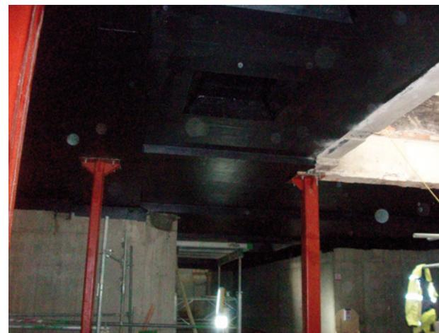
*TT Vapour Membrane provides a water and gas proof barrier to new soffits*
