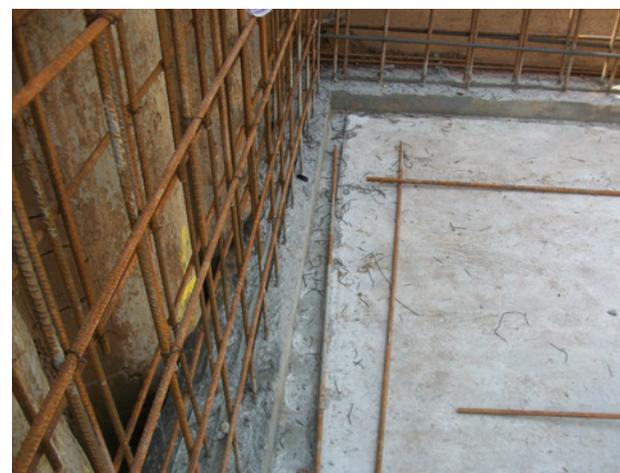
Pre-formed recess in floor slab to accept TT Waterstop
