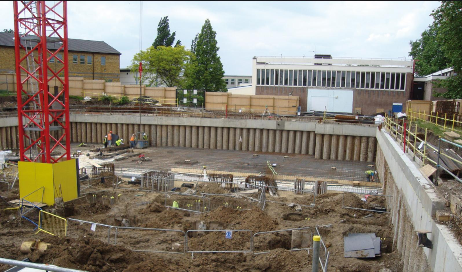
*The first of three pours in the construction of the watertight concrete floor slab*
